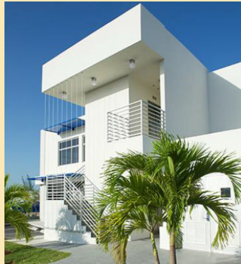
SWP's secure storage facility George Town, Grand Cayman
